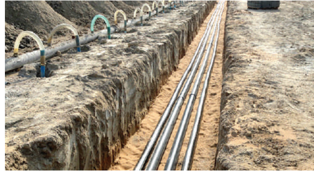
33 KV CABLE LAYING
