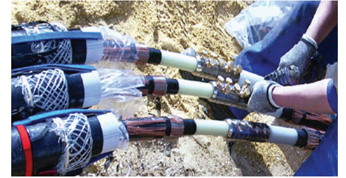
33 KV CABLE JOINTING
